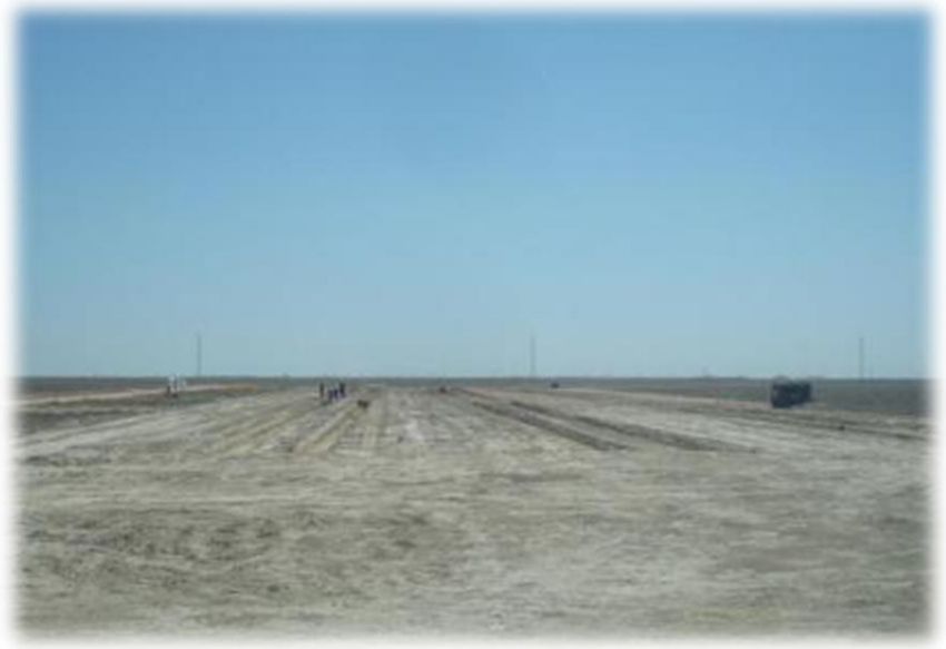
Photo 2: Tree Nursery Surface Leveling
